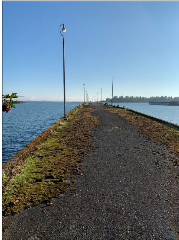
Photograph 11. Pier 6, deck Looking east
