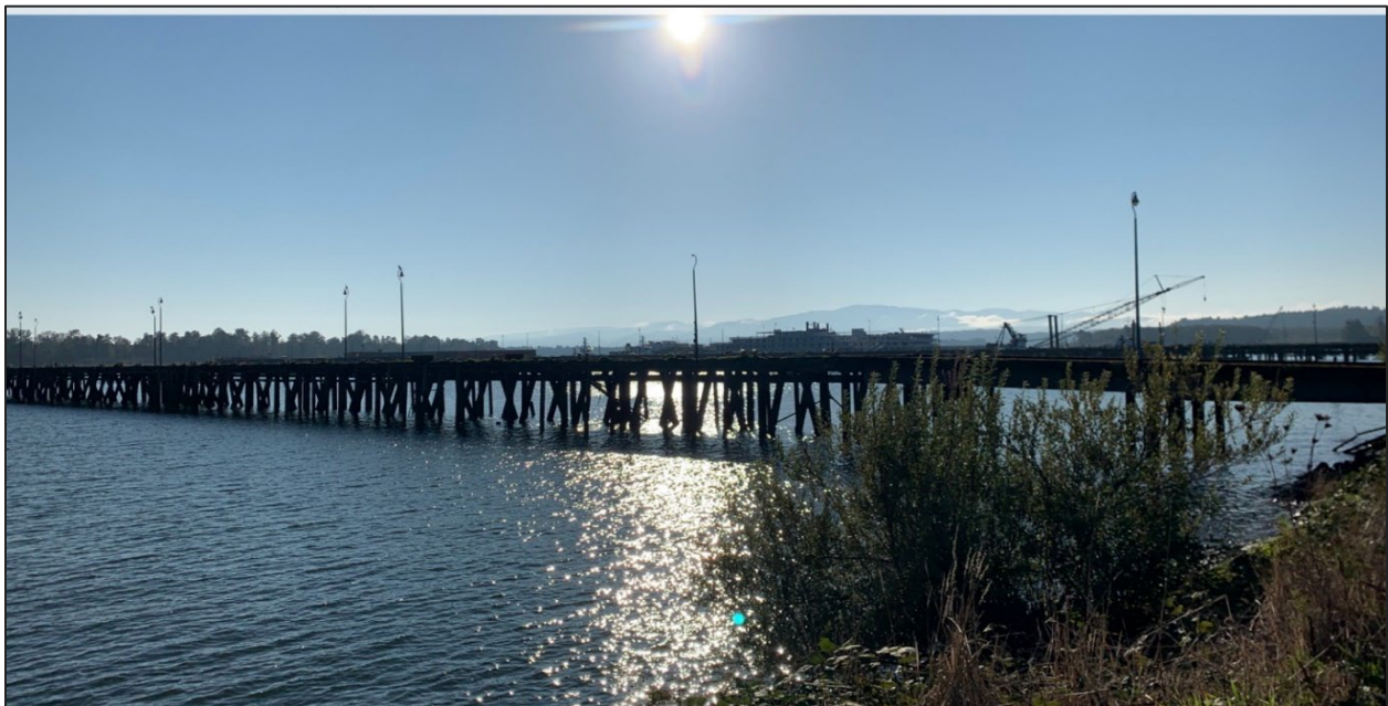
Photograph 12. Pier 6, north side Looking southeast
