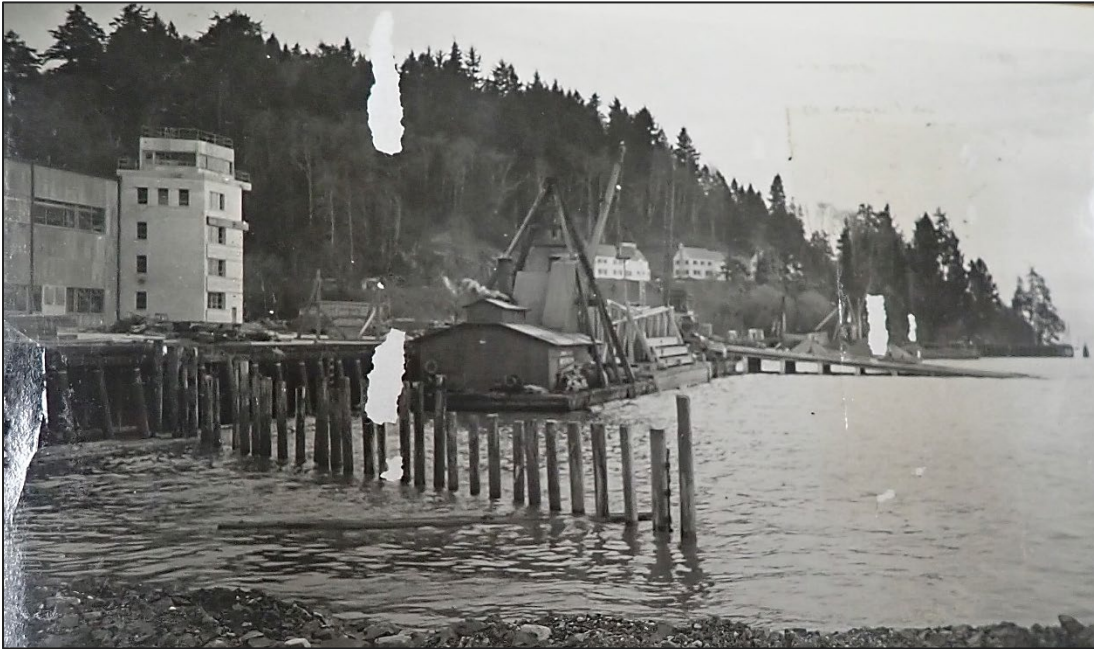
Photograph 3. Dock and ramp from new fill, looking northwest, February 1941 (Photo on file at DOL)
