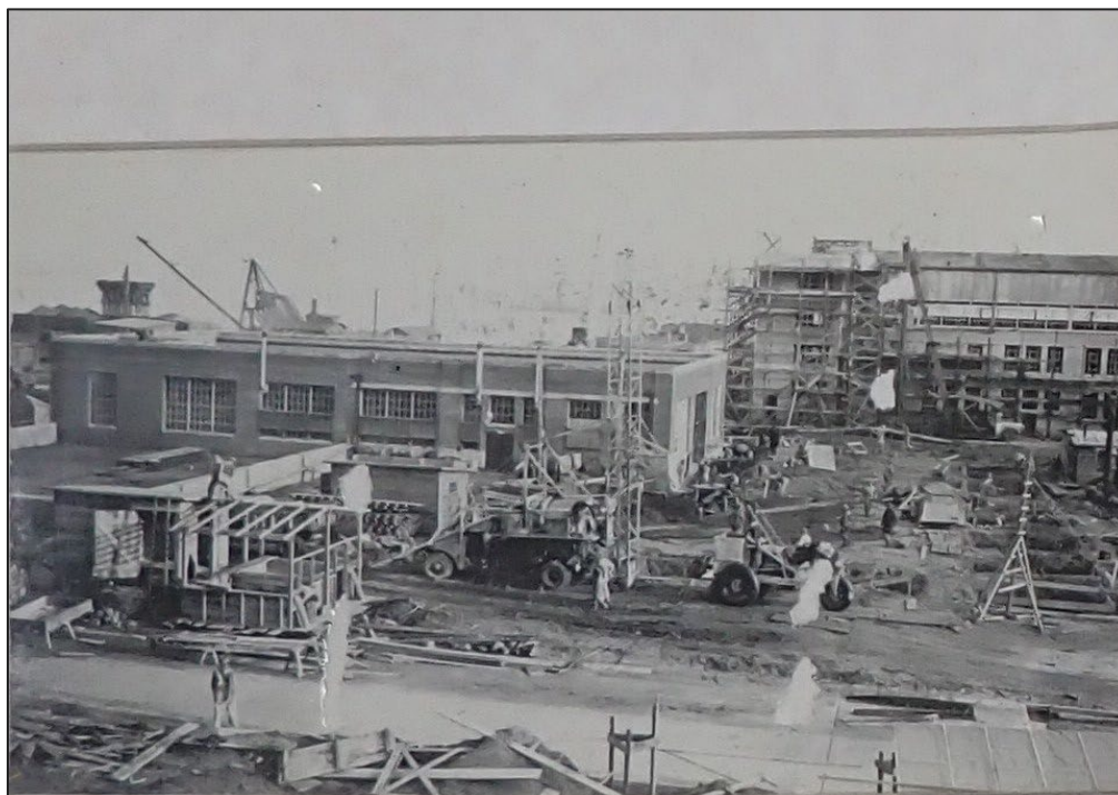
Photograph 5. Construction of NAS Tongue Point, looking west, c. 1940 (Photo on file at DOL)
