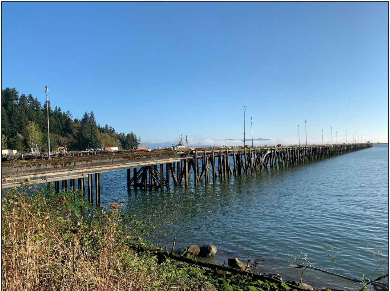
Photograph 10. Pier 6, south side Looking northwest
